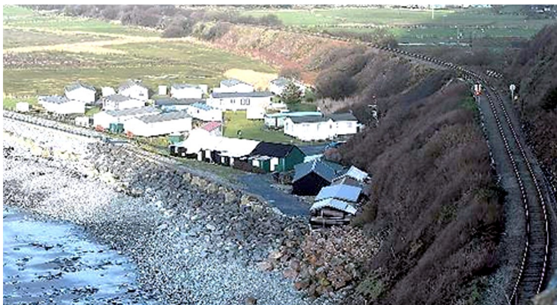
Figure 10: Repairs to the coastal defences at Friog corner, carried out in the 1990's. These works included the placement of rock armour along the line of the sea wall.
