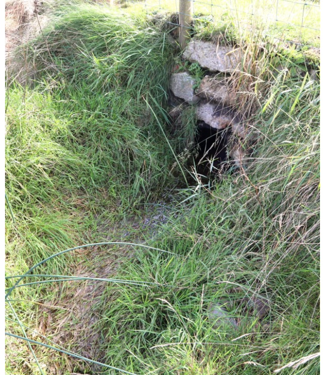
Figure 26: (left) drainage ditch constructed in front of the caravan park to intercept groundwater flow through the shingle spit at high tide. (right) culvert discharging into the Friog drainage ditch network.
