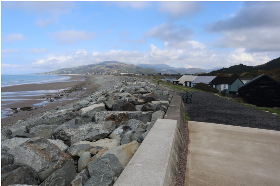
Figure 17: Replacement section of concrete sea wall in the foreground, with rock armour.
