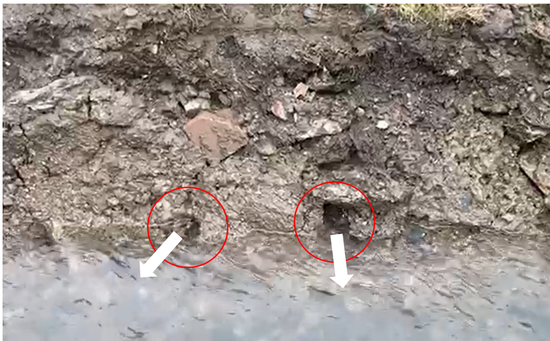
Figure 27: Groundwater seen to be flowing out of soil pipes (ringed in red) into the drainage ditch at the northern end of the caravan park..
