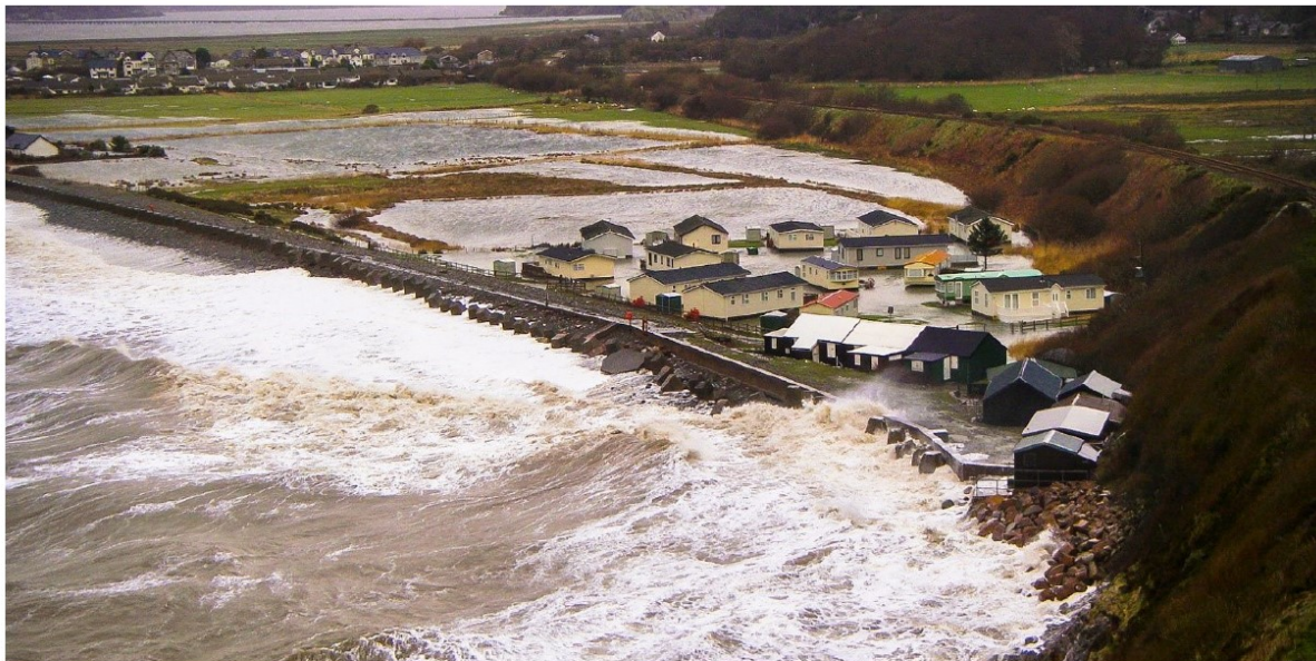
Figure 1: Failure of the eroded section of the Ro Wen shingle spit at Friog corner during a storm, causing localised flooding.
