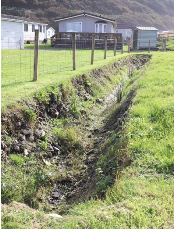
Figure 26: (left) drainage ditch constructed in front of the caravan park to intercept groundwater flow through the shingle spit at high tide. (right) culvert discharging into the Friog drainage ditch network.
